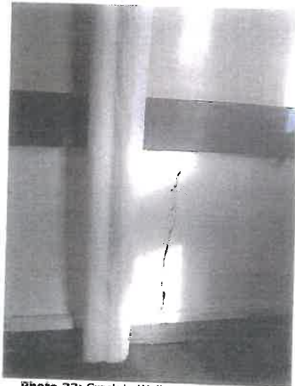
Photo 33: Crack in Wall at Front Entrance
