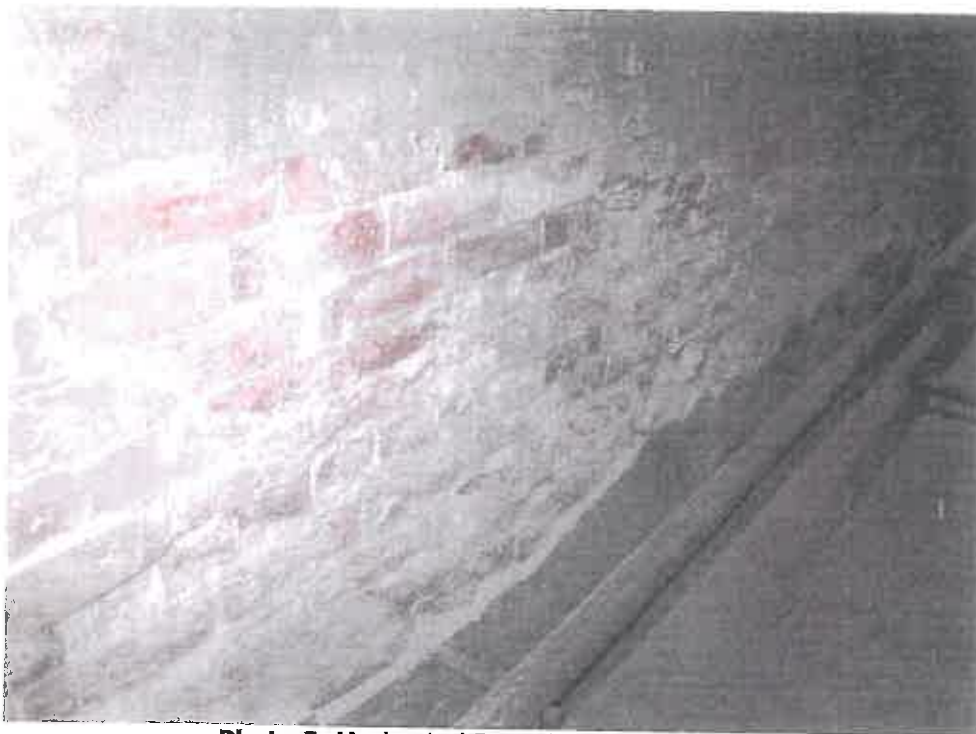
Photo 2: Mechanical Room Wall Deterioration
