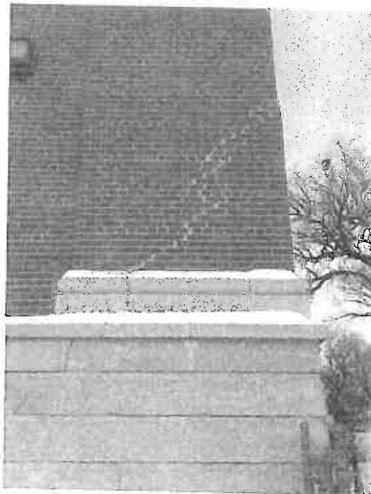
Photograph 12: Existing crack on the southeast exterior wall.
