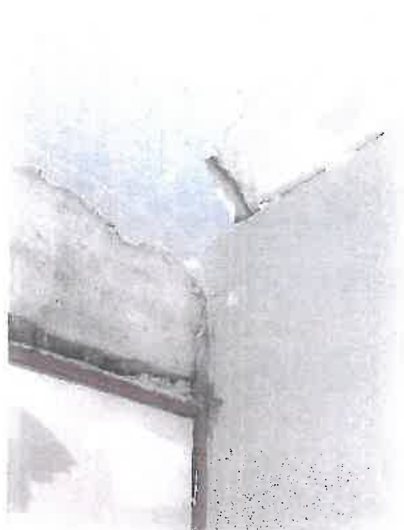
Photo 23: Cracking in Beam and Slab
