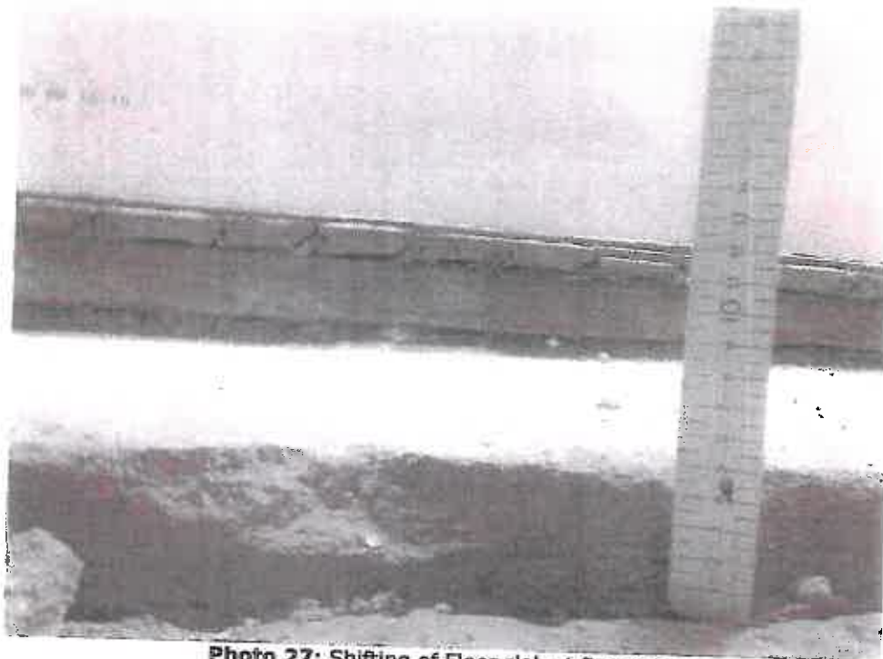
Photo 27: Shifting of Floor slab at Room 12
