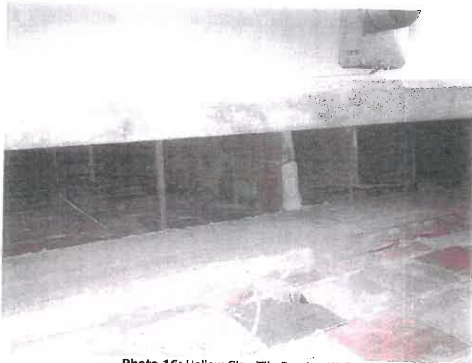
Photo 16: Hollow Clay Tile Bracing Wall
