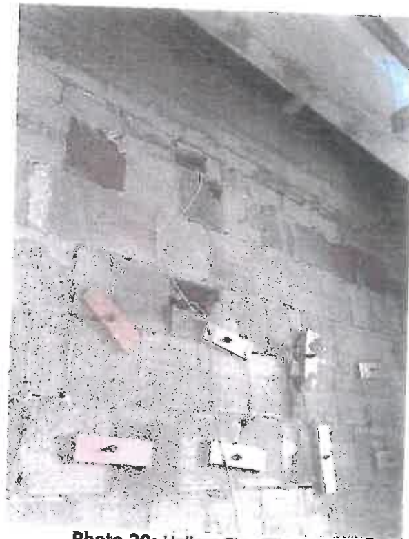
Photo 29: Hollow Clay Tile Wall
