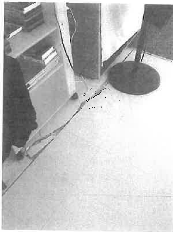
Photo 2: Wise Owl Daycare- Cracks in concrete at heave location
