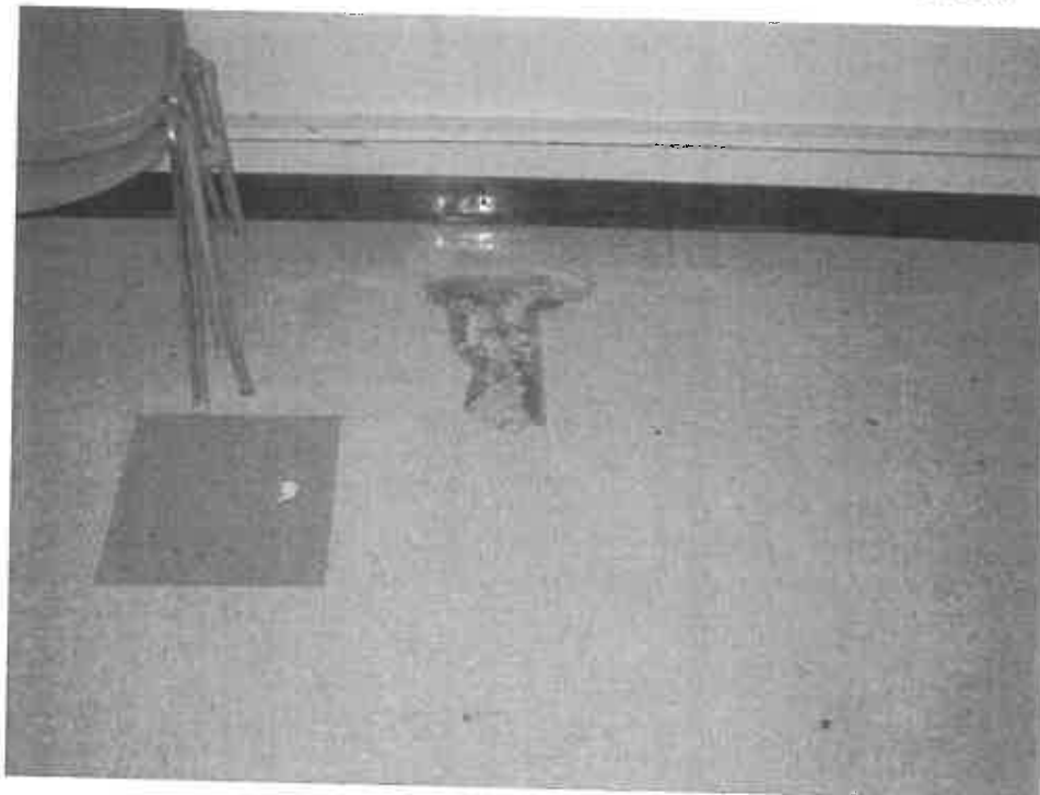
Photograph 02: Broken floor tile in Room 8 of the basement floor.
