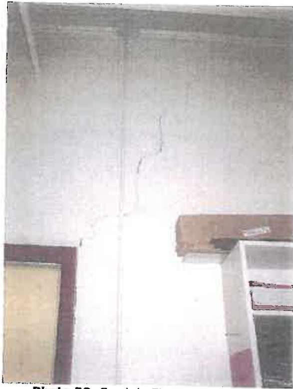
Photo 30: Crack in Storage Room Wall
