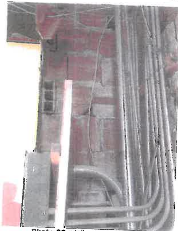
Photo 28: Hollow Clay Tile Wall
