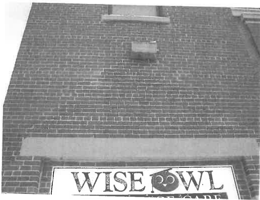
Photograph 10: Re-cracking of the mortar in the wall above the southwest entrance.
