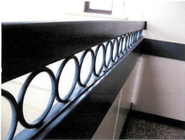
Hardwood handrails and ironwork, north and south interior stairs.
