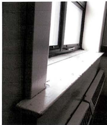
Original window casings.
