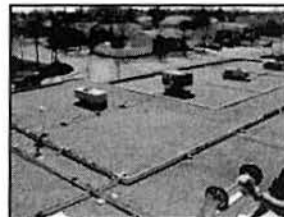
Buck - View from Gym Looking SW.jpg
