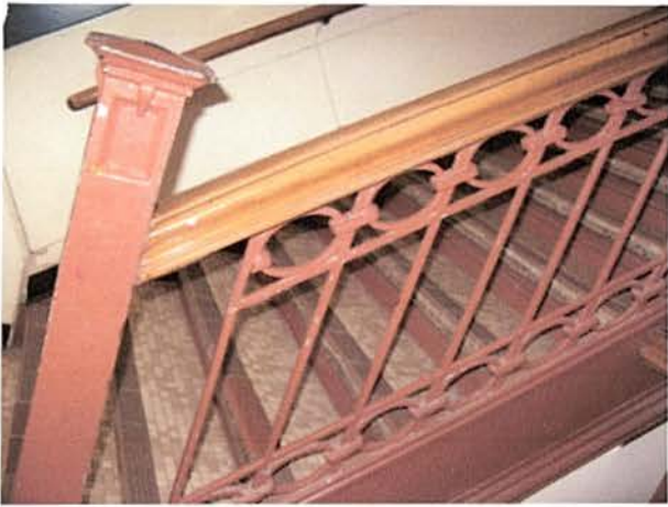
Hardwood handrails and ironwork, north and south interior stairs.
