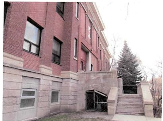
Staircase and stone base, showing original window recesses.
