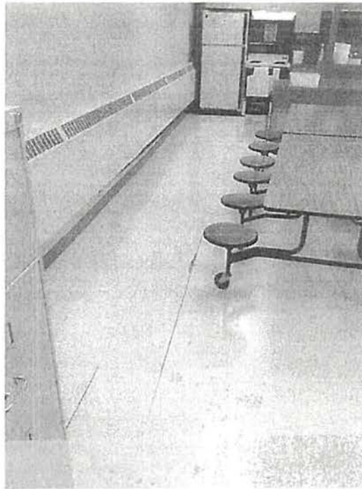
Photo 1: Nutrition Room- Cracks in tile at floor heave location
